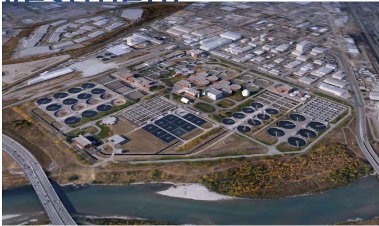
Bonnybrook WWTP expansion
