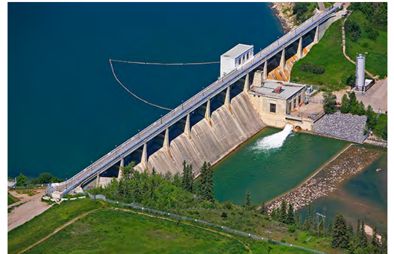
Glenmore WTP upgrades
